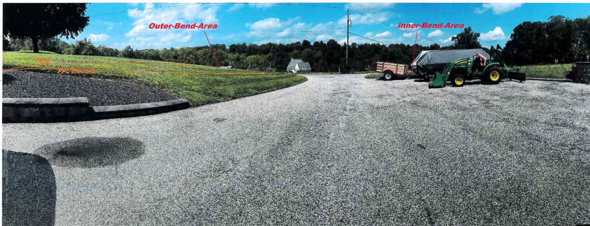
706 Callowhill Rd_View away from House
